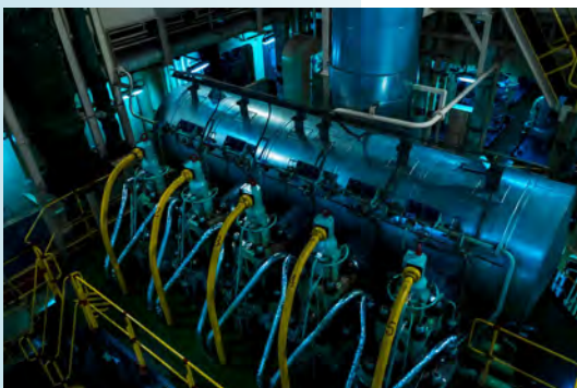
Machinery Status Alerts
